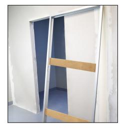
G. Insert the assembled door frame into the finished construction opening
