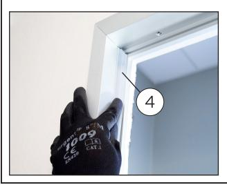
P. Place the seal [4] in the seat by trimming it appropriately in the door frame corners and to the profile length
