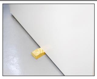
R. Place the door onto the door frame by lifting it using the wedge inserted under the door, which facilitates fixing the door on the hinges
