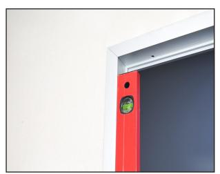
K. Insert the door frame into the construction opening again in such a way that the places for hinges are aligned with those cut out in the wall. Again check the vertical and horizontal placement.
