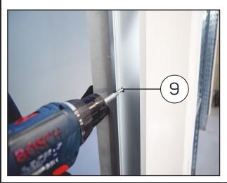
L. Using screws [14] tighten door frame profiles to the wall structure (in the case of a masonry opening - use expansion bolts [15])
