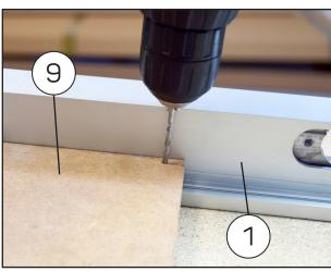
D. Add expansion strips [9] to the door frame and drill holes for screws in the expansion strip at the height of the seal seat, making sure that the door frame profile is not pierced [1]
