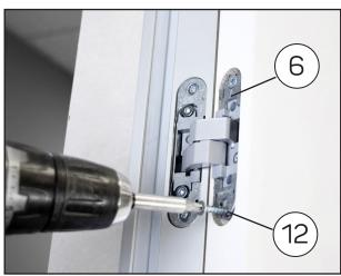
S. Screw the hinges [6] to the door after pre-drilling holes for screws [12] to prevent delamination of door stile
