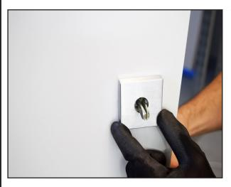
T. Place the door rosette and the door handle spindle
