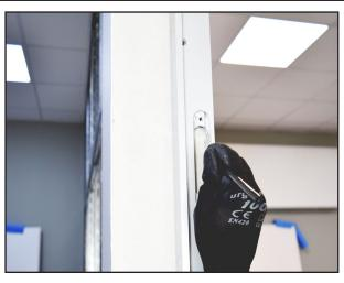
Draw the places of hinge installation on the wall, and then temporarily remove the door frame from the construction opening
