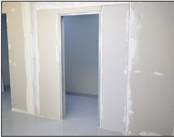
2E. Door frame with plasterboard built over it
