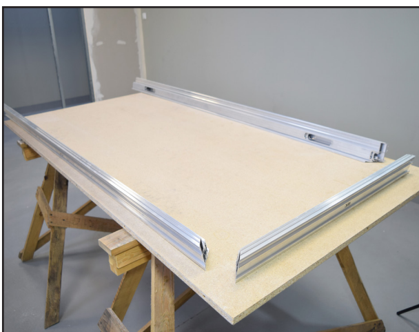
B. Spread the door frame profiles
