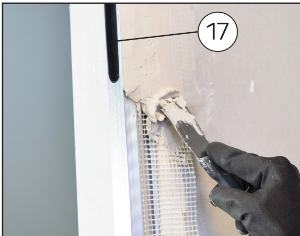
2F. Insert the plastic caps [17] into the hinge seats. Fill in jointing of plasterboard and door frame with plaster and reinforce it with a glass fibre mesh to join the panels
