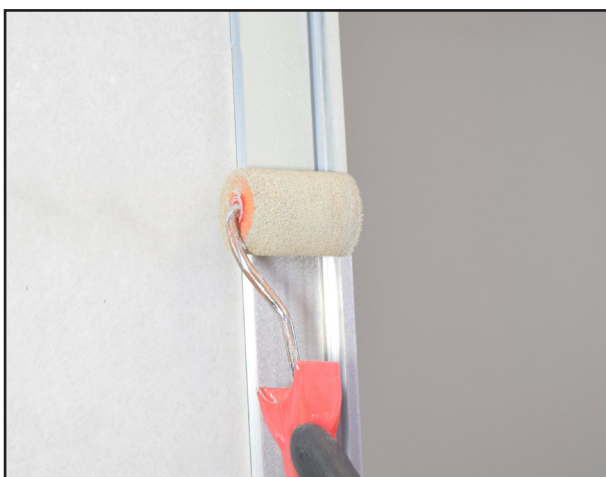
2H. Paint the surface of the profiles using aluminium primer [18], and after it has dried completely, paint the door frame with a wall paint. When painting, use covers for hinge stiles [16] and the hinges [17]
