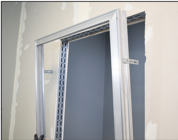
N. Insert the assembled door frame into the construction opening
