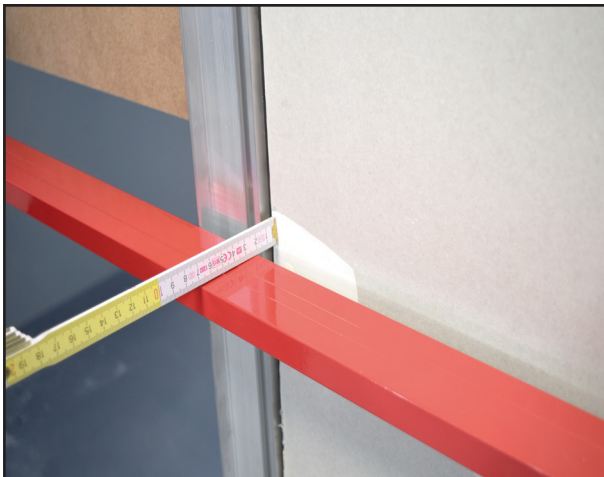
O. Pay particular attention to the door frame bite. The outer edge of the door frame should protrude in relation to the opening by the thickness of the lining placed later on the wall
