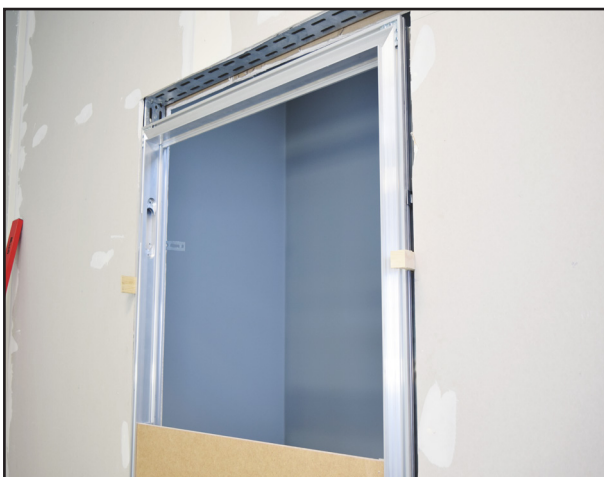
P. Then wedge the door frame in the opening
